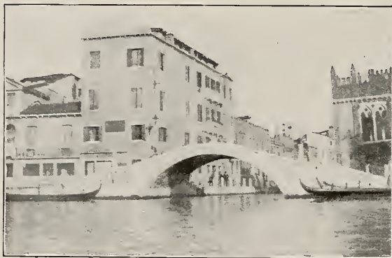
A TYPICAL BRIDGE, VENICE.
